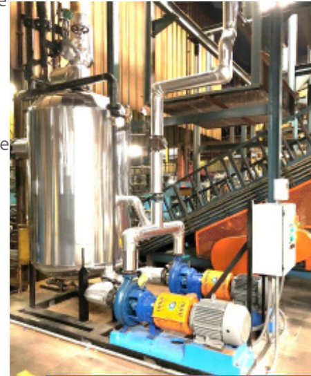
Figure 4: Electric Continuous Flow Pumping Unit
