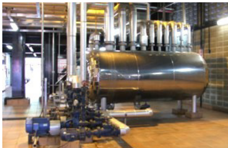
Figure 1: New Condensate Tank Installation
