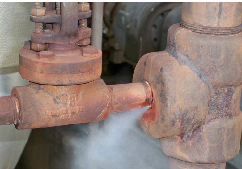
Figure 3: Corrosion Resulting in Steam Leakage
