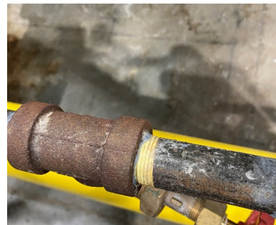
Figure 9: NPT Installation
