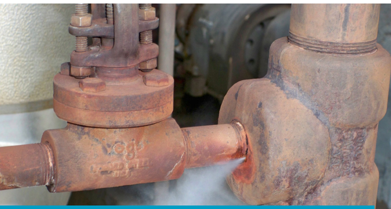
Figure 11: Thread Failure and Leakage
