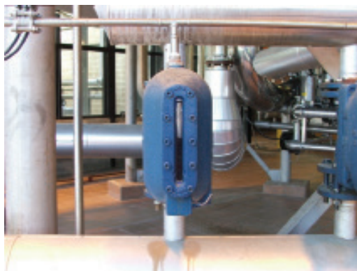
FIGURE 1. Shown here is a visual indicator on a steam trap
