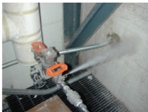
FIGURE 2. A steam trap test valve is shown here
