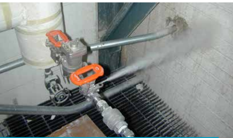
Figure 2: . Flash Steam and Condensate Discharging From a Steam Trap Test Station
