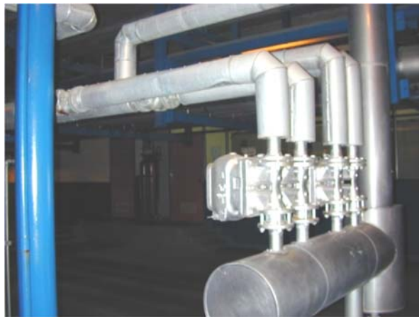
Figure 3. Connecting Into the Condensate Header
