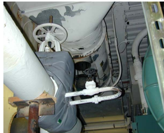
Figure 10. Isolation Valve Purchased With a Warm-Up Valve and Loop
