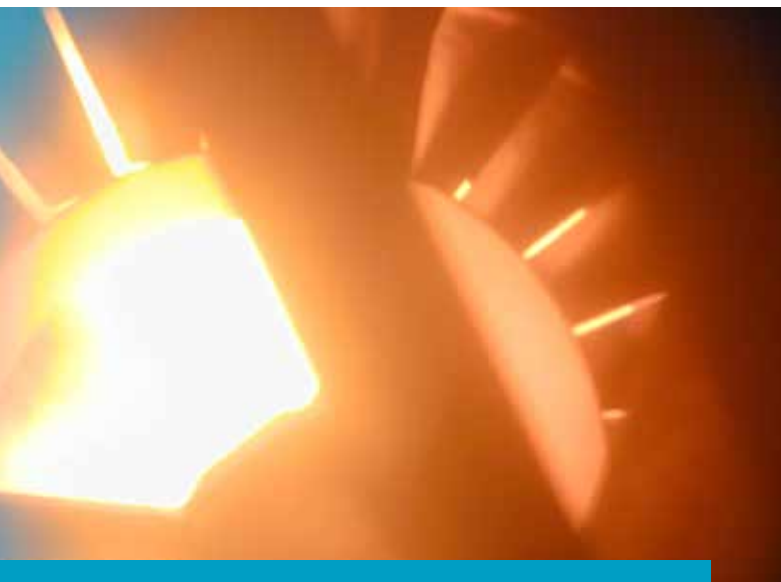
Figure 1: Natural Gas Burner in Operation
