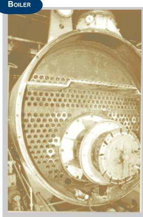
The boiler failed after 6 years even though its normal life expectancy is 20 to 30 years. Because the repair costs \$23,800, preventing early failures decreased yearly repair costs by 70% (from \$3,967 per year to \$1,190 per year).
