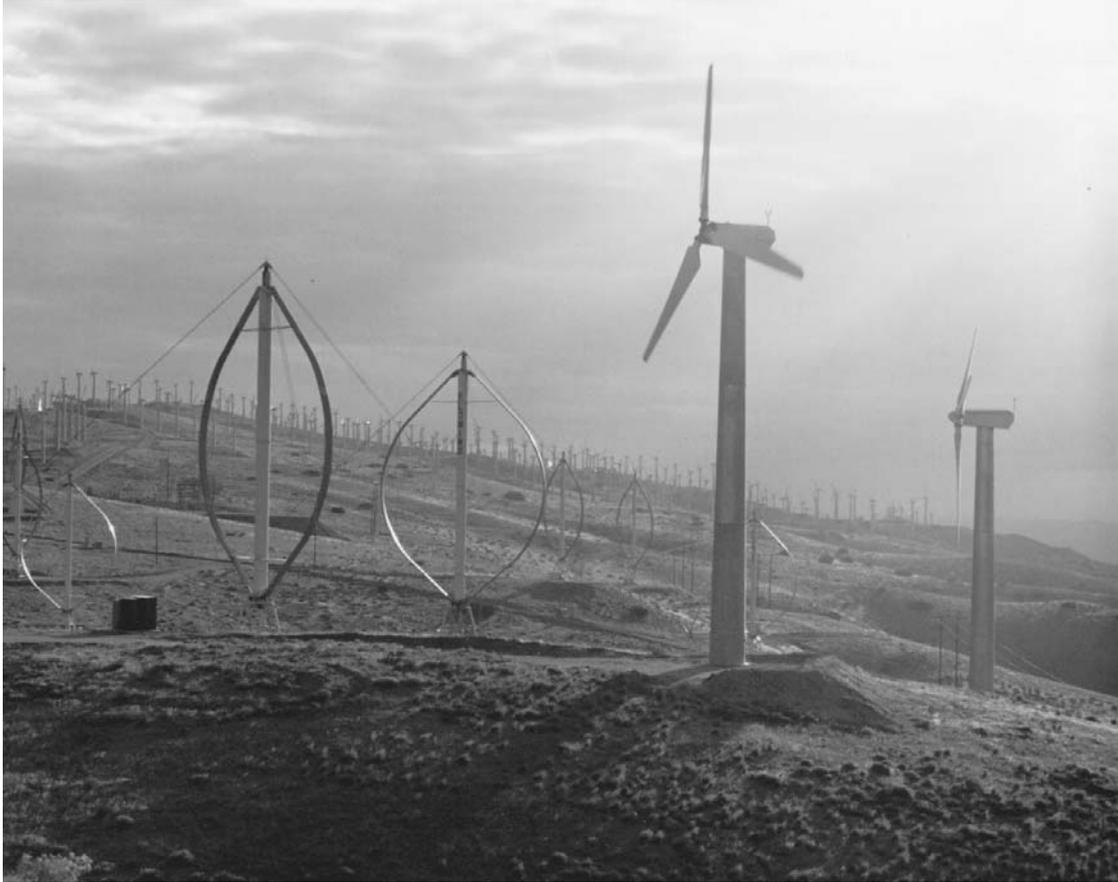
**FIGURE 8.11.2** Wind farm both horizontal-axis and vertical-axis turbines.
