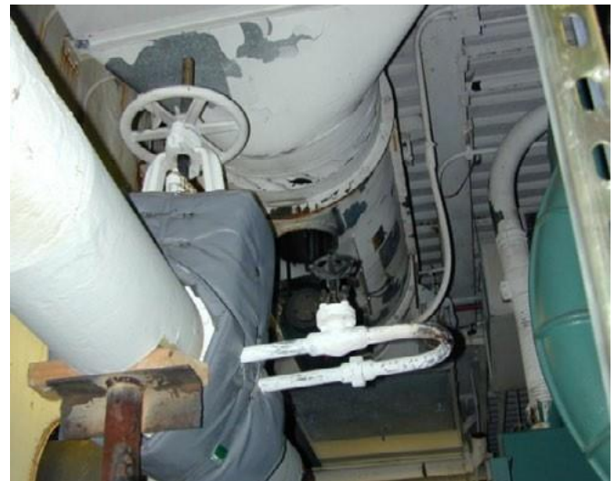
Figure 3: Isolation Valve with a Warm-Up Loop
