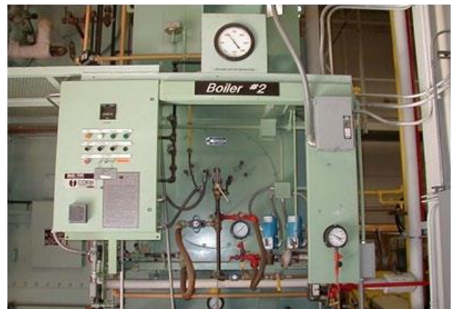
Figure 3: Natural gas/fuel oil burner
