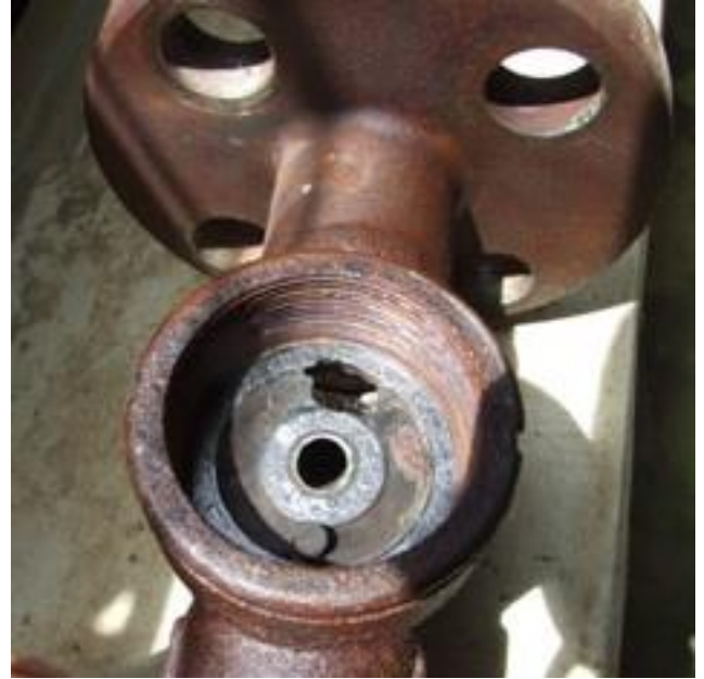
Figure 4: Visual failure inspection STEAM TRAP STATION EVALUATIONS
