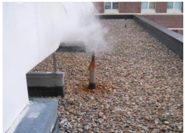
Figure 2: Steam venting due to steam trap station failure
