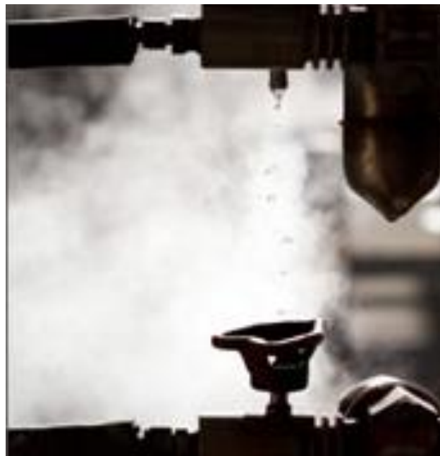
Figure 3: Visual testing for steam traps
