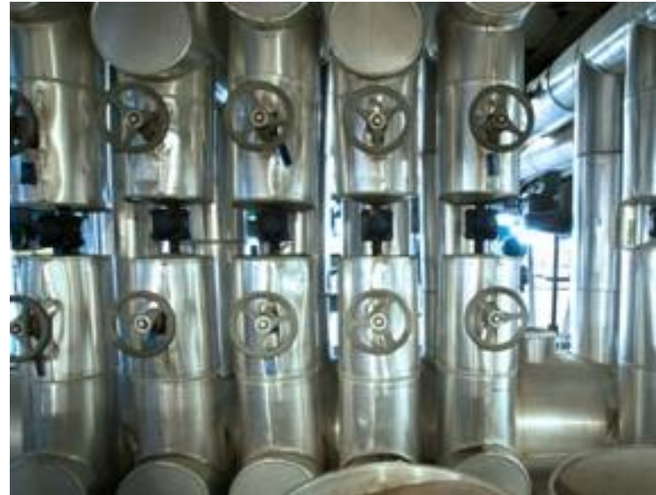
Figure 1: Steam Trap Station Installation
