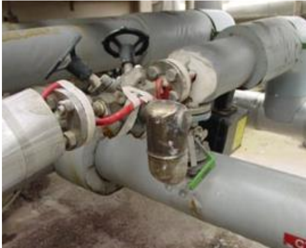
Figure 6: Steam trap station with universal connector and isolation valves
