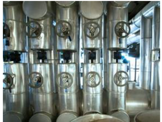
Figure 1: Steam Trap Station Installation
