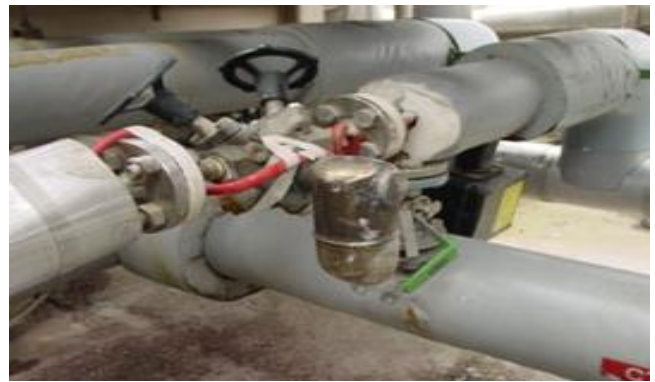
Figure 5: Steam Trap Station with Universal Connector and Isolation Valves
