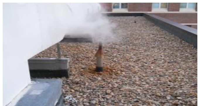
Figure 2: Steam venting due to steam trap station failure
