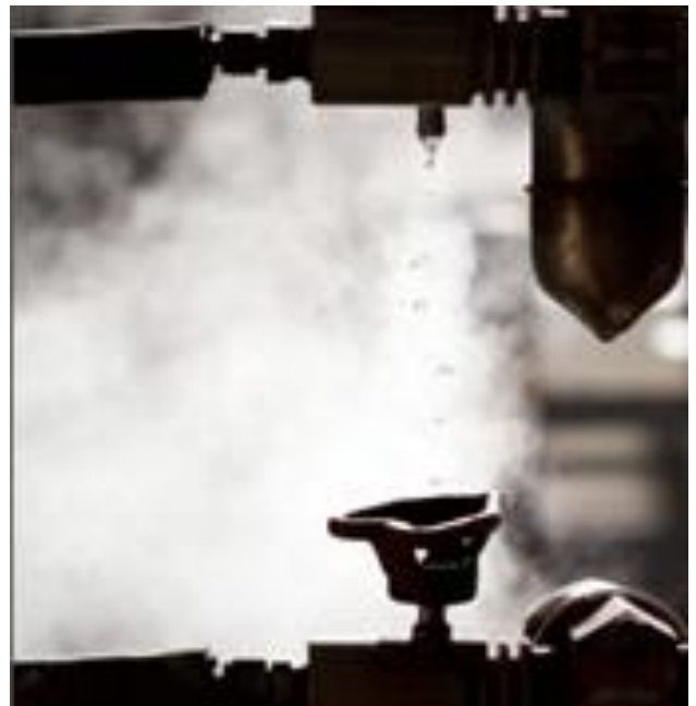
Figure 3: Visual Testing for Steam Traps
