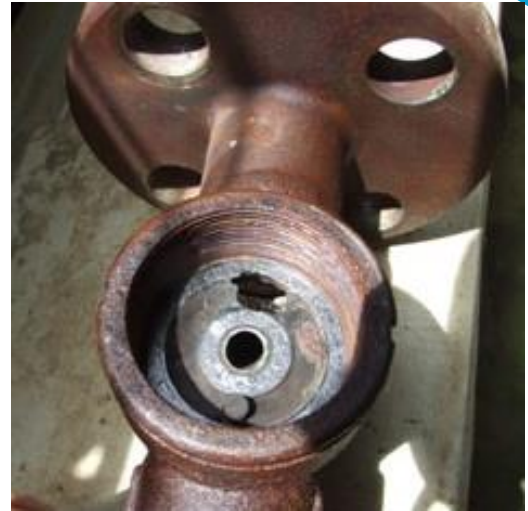
Figure 4: Visual Failure Inspection
