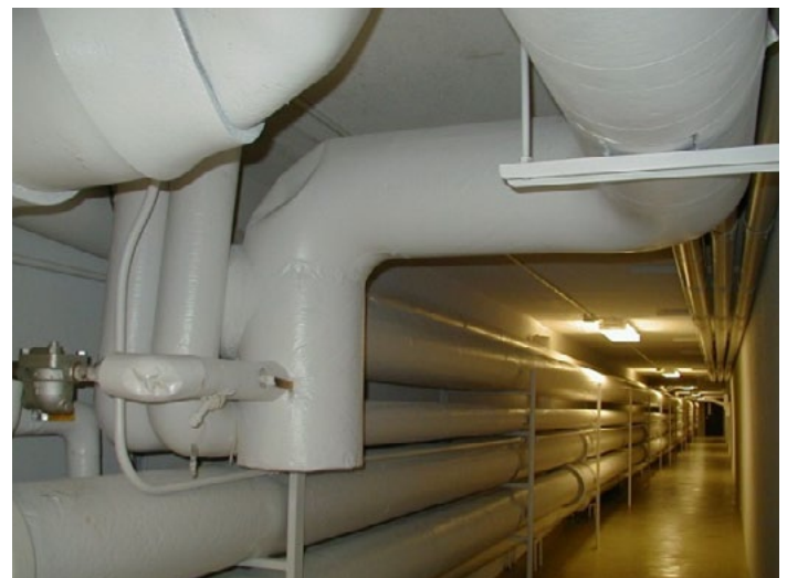
Figure 2: Steam Distribution System
