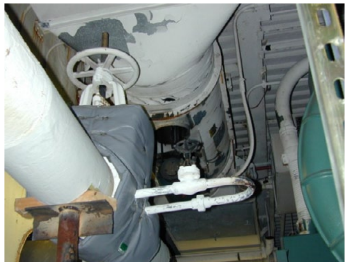
Figure 3: Isolation Valve with a Warm-Up Loop
