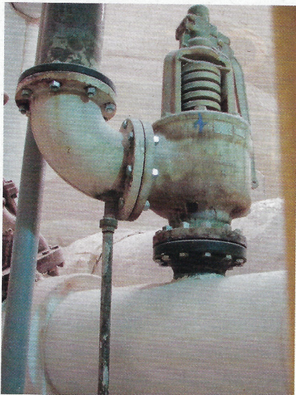
FIGURE 6. In this photo, the discharge vent line is attached directly to the safety valve, which is an incorrect configuration that can result in excess stress being placed on the valve body
