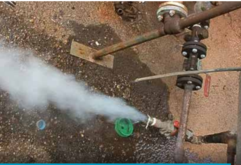
Figure 3: Unacceptable Steam Quality
