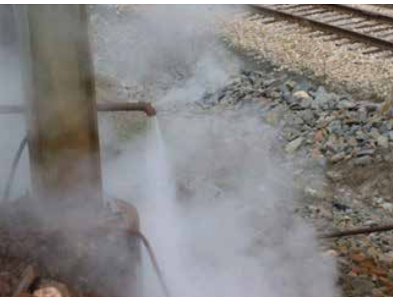
Figure 4: Unacceptable Steam Quality
