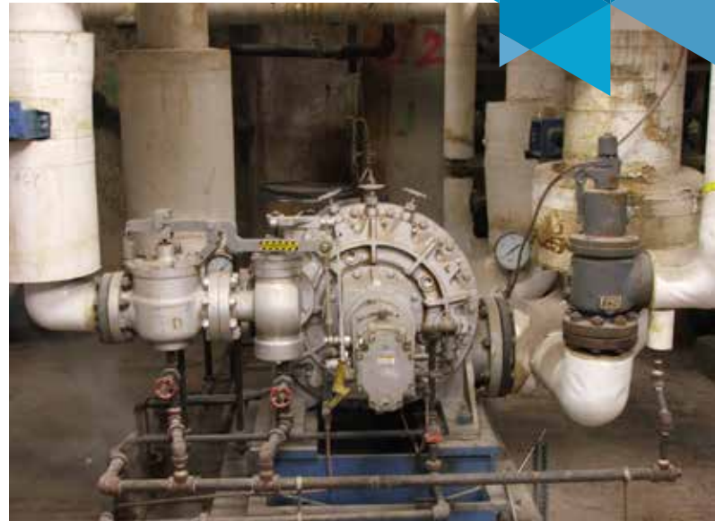
Figure 4: Small Steam Turbine Installation
