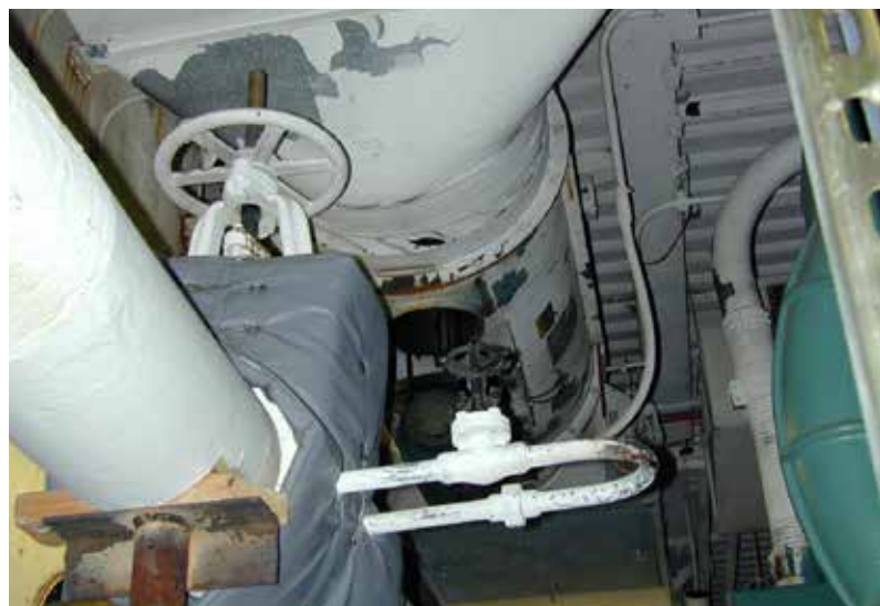
Figure 4: Warm-Up Valve Built Internally into the Valve
