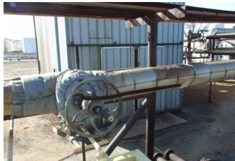
Figure 2: Isolation Valve: External Force Being Applied by a Bar to Open
