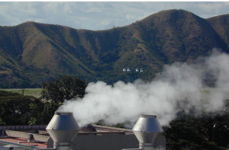
Figure 1: Flash Steam Losses
