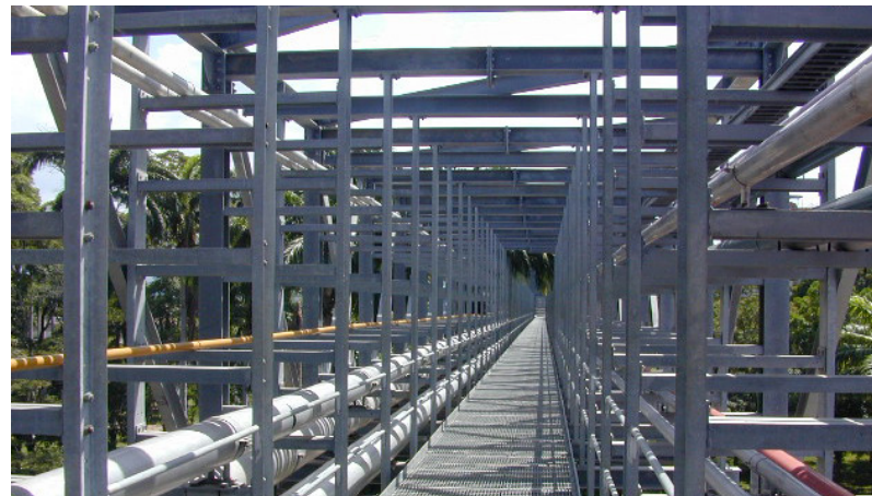
Figure 4: Condensate Line Installation
