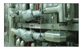
A proactive insulation-management program is critical to overall steam system thermal-cycle efficiency. Furthermore, because steam systems operate above 212°F (100°C) and as high as 1200°F (649°C), the negative effects of uninsulated components can be dramatic and are unacceptable in today's industrial steam system operation.
