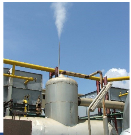
Figure 7: Deaerator Venting
