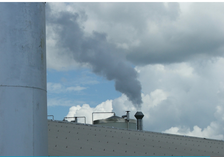
Figure 6: Steam Venting From an Unbalanced Steam Header
