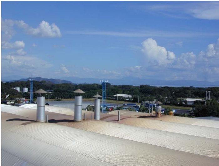
Figure 12. Plant Operation: No Steam Venting
