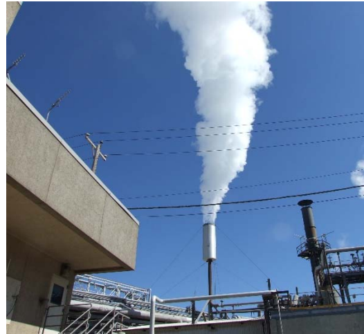
Figure 3. Flash Steam Venting
