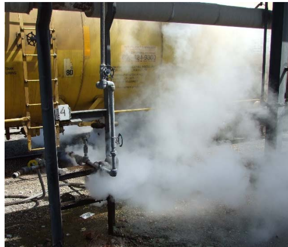
Figure 26. Threaded Connection Leakage
