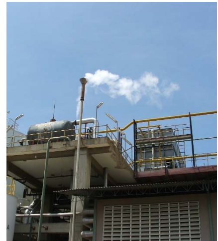
Figure 4. Flash Steam Venting to the Atmosphere
