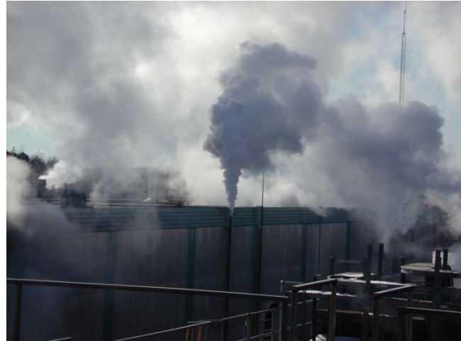
Figure 2. Example of an Unbalanced Steam System
