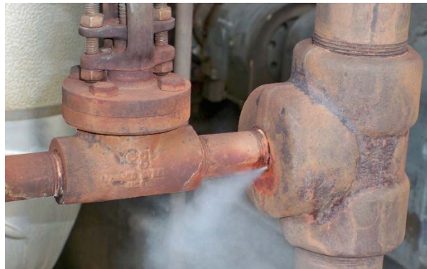
Figure 25. Steam Leakage at a Connection
