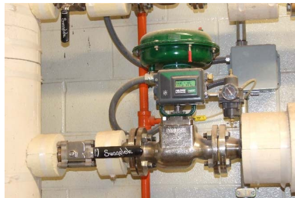
Figure 32. Steam Isolation Ball Valve Before the Control Valve
