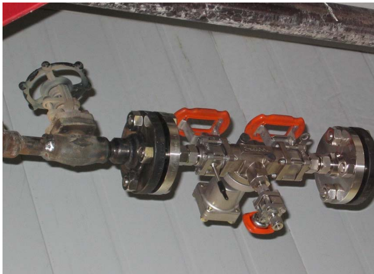
Figure 30. Welding and Flanges for a Leak Free Connection
