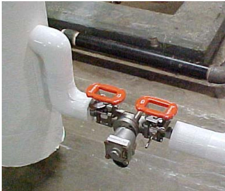
Figure 31. Swagelok Tube Connectors for a Typical Steam Trap Station Installation for a Leak-Free Operation
