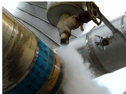
Figure 27. Internal Valve Leakage
