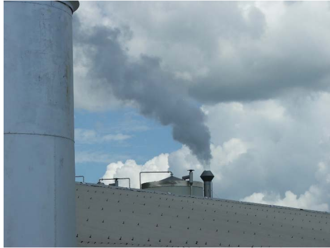
Figure 6. Steam Venting From an Unbalanced Steam Header
