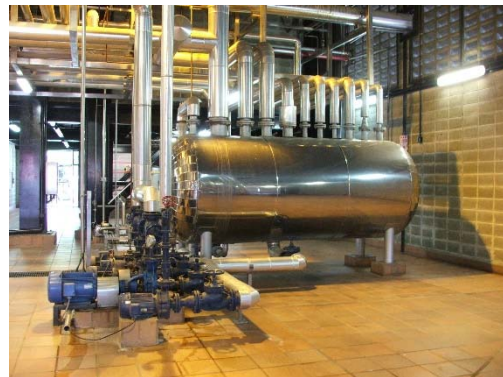
Figure 13. New Pressurized Condensate Tank System
