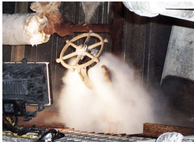
Figure 28. Valve Packing Leakage
