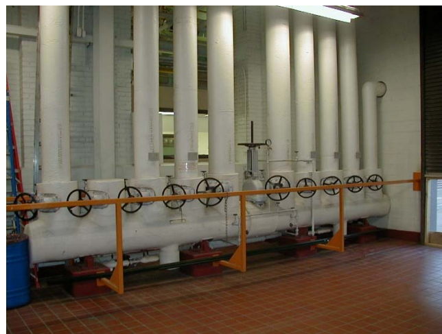
Figure 29. Leak-Free Steam System
