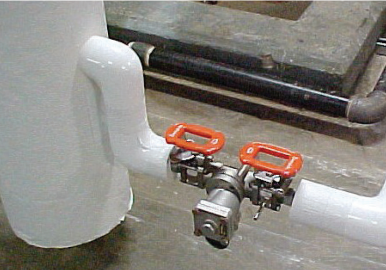
Figure 7: Swagelok Tube Connectors for a Typical Steam Trap Station Installation for a Leak Free Operation
