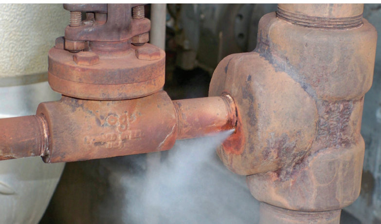
Figure 1: Steam Leakage at a Connection
