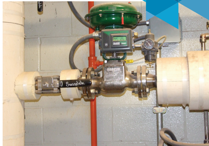
Figure 8: Steam Isolation Ball Valve before the Control Valve
