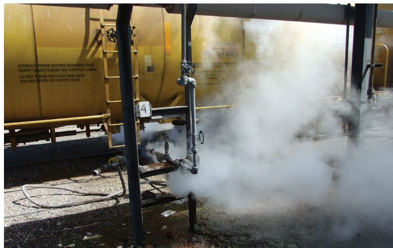
Figure 2: Threaded Connection Leakage
