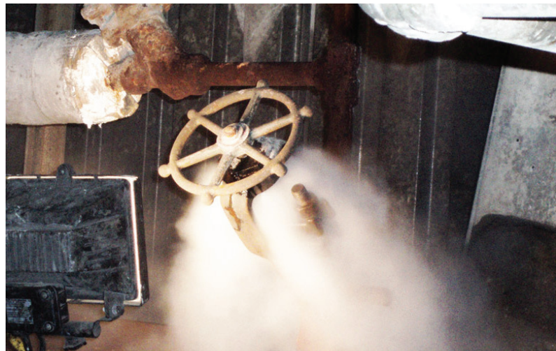
Figure 4: Valve Packing Leakage
