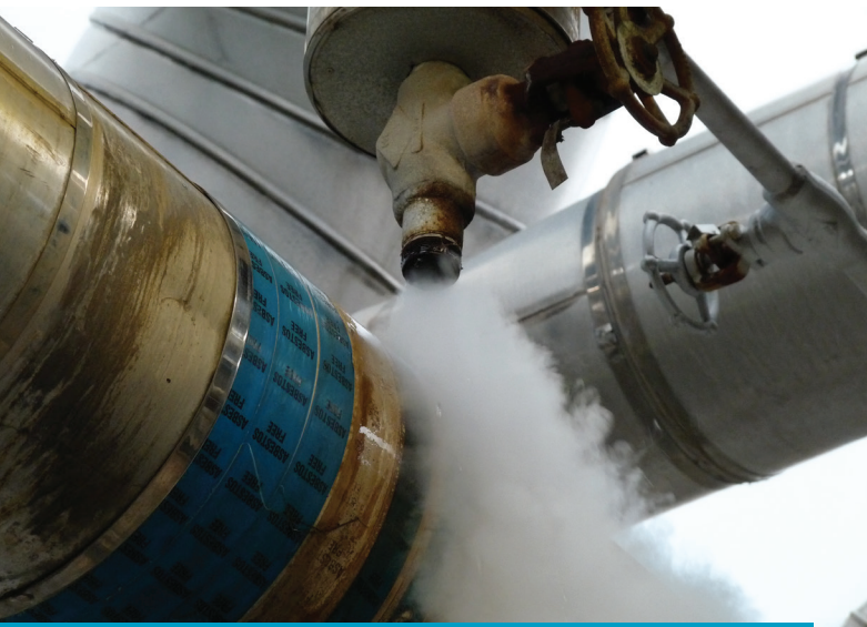
Figure 3: Internal Valve Leakage
