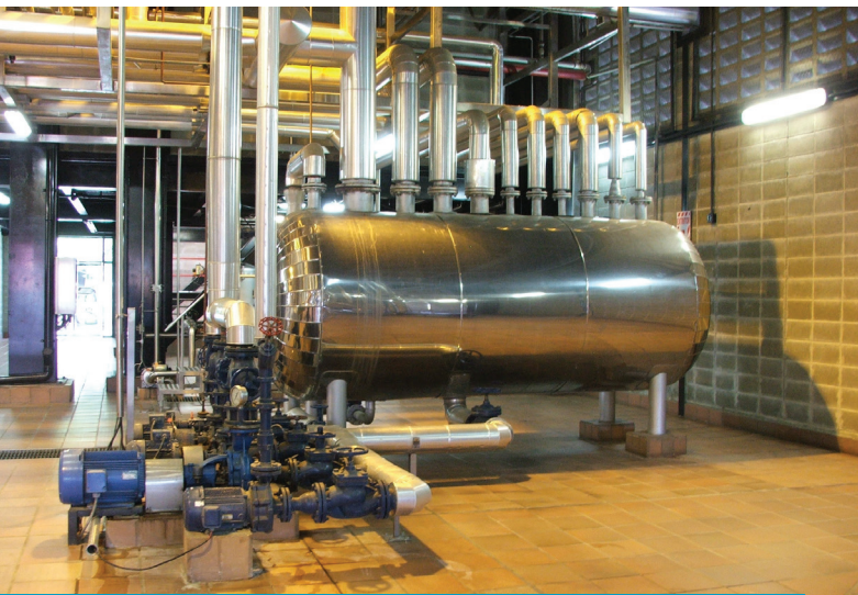
Figure 1: New Pressurized Condensate Tank System
