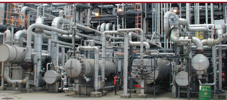
Figure 2. Heat Exchangers in a Process Plant
