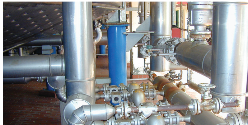
Figure 5: Flow Indicators Installed
