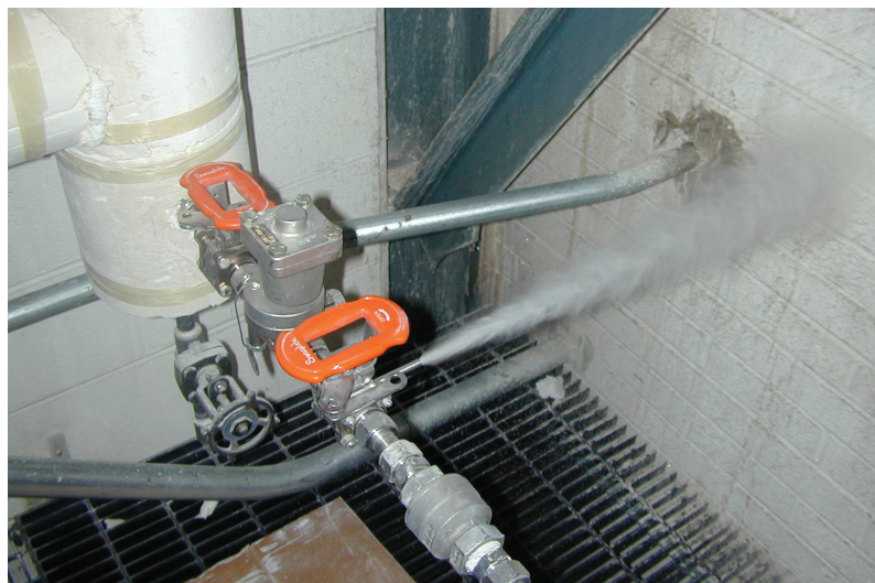
Figure 2: Steam Trap – Discharging Flash
